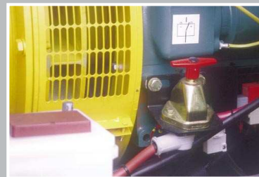
Battery cut-off-switch
