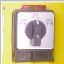
Voltage selector switch
