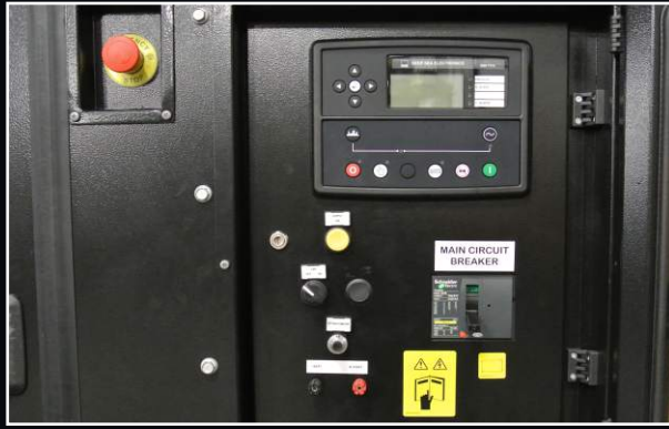
Control panel, with Deep Sea Controller, laid out and labeled for easy use.
