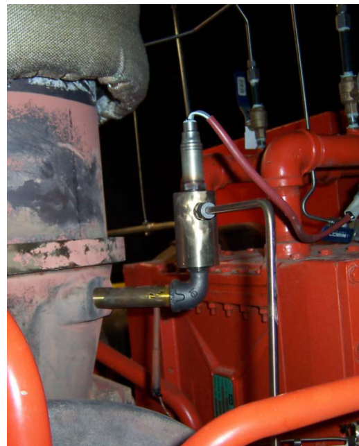
Illustration 9 – Correct installation - HEGO Sensor is mounted in the 12:00 o'clock position
