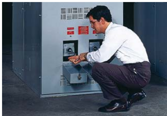
Figure 26: External Manual Operator (EMO) Operation
