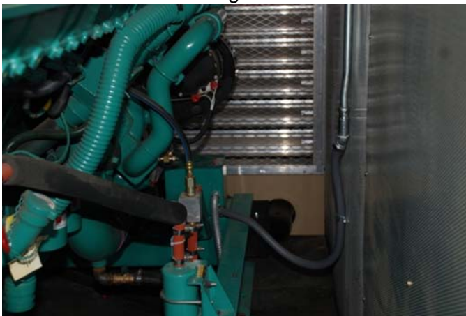
Engine Water Jacket Heater
